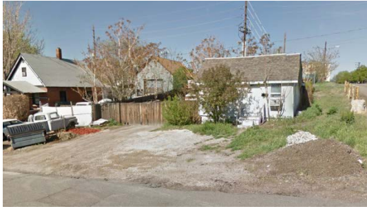
Subject site, looking west.
