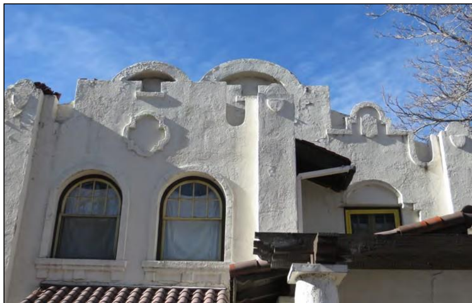
Photograph 2 (right): East side close-up of shaped parapet and arched windows
