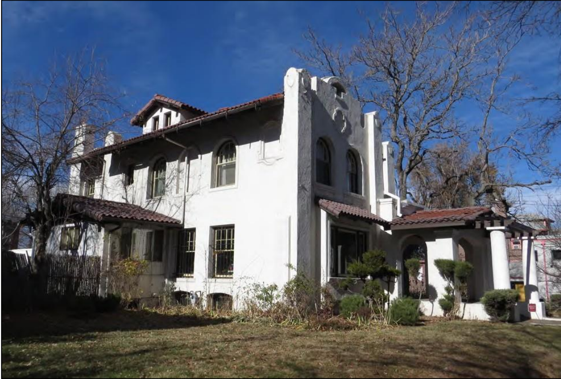
Photograph 3 (above): South side of house
