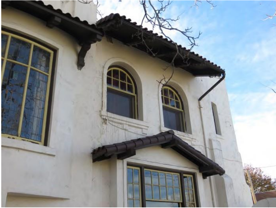
Photograph 7 (left): North side close-up of overhanging eaves and arched windows
