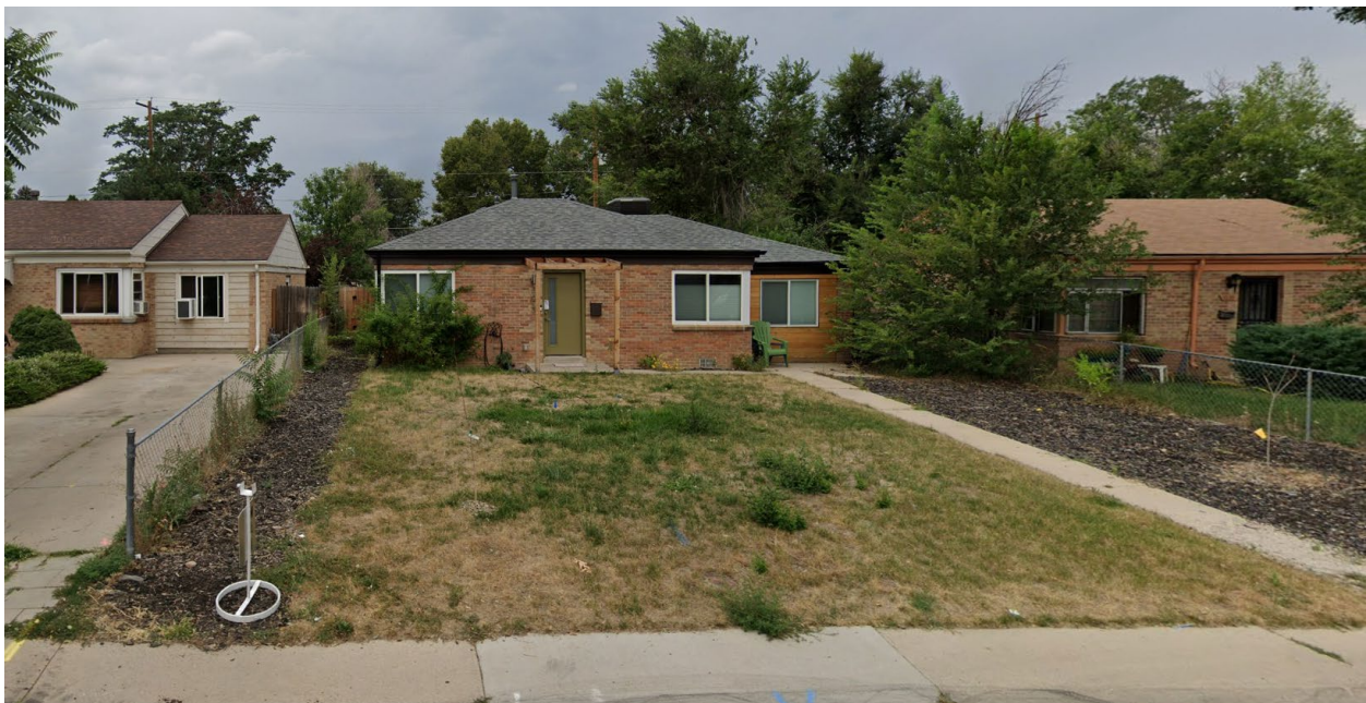
View of the subject property looking west.
