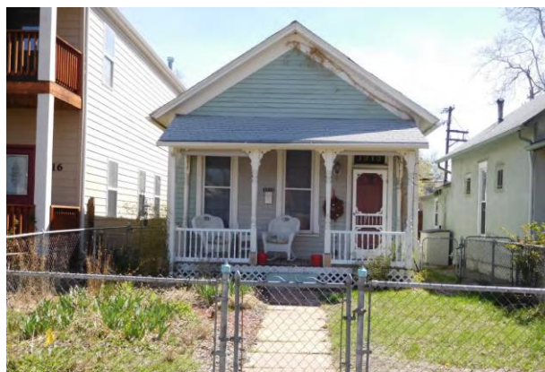
Structure in proposed district, example of an Italianate Cottage
