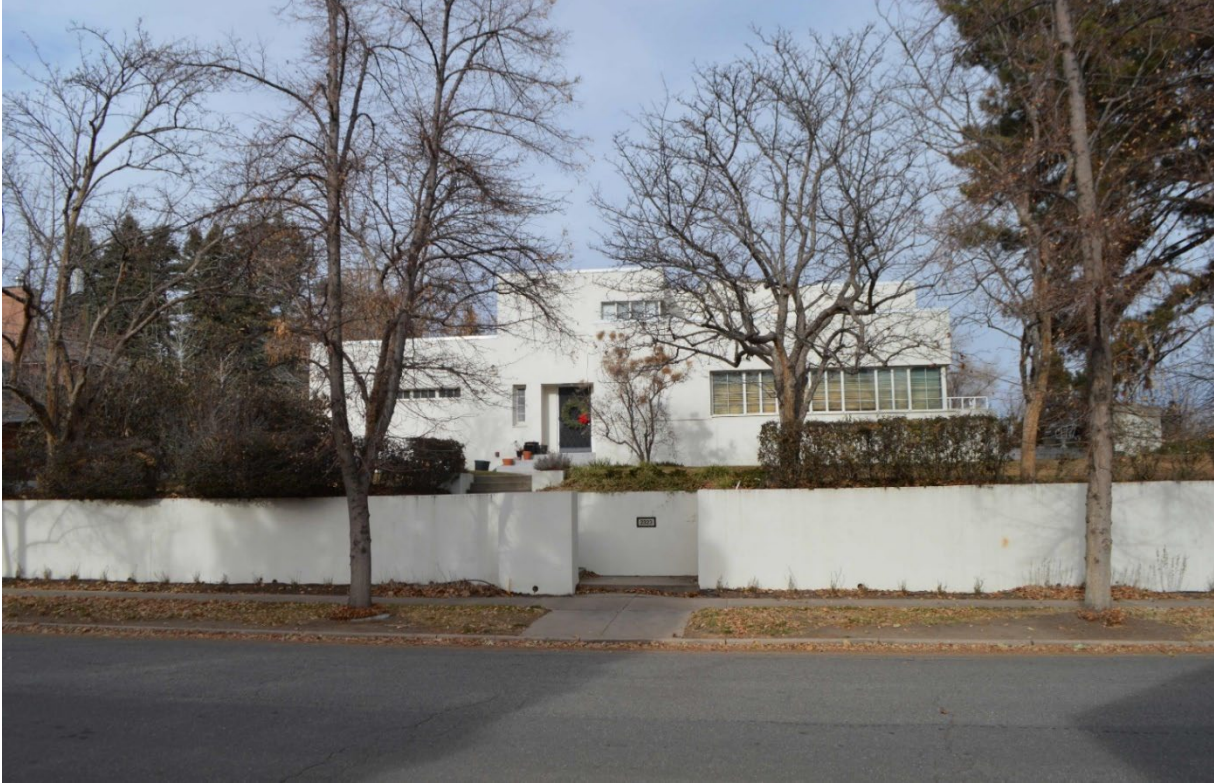
1. Front of the house from East Dakota Avenue. Photographer: Thomas H. Simmons. Date: December 2022. View north.
