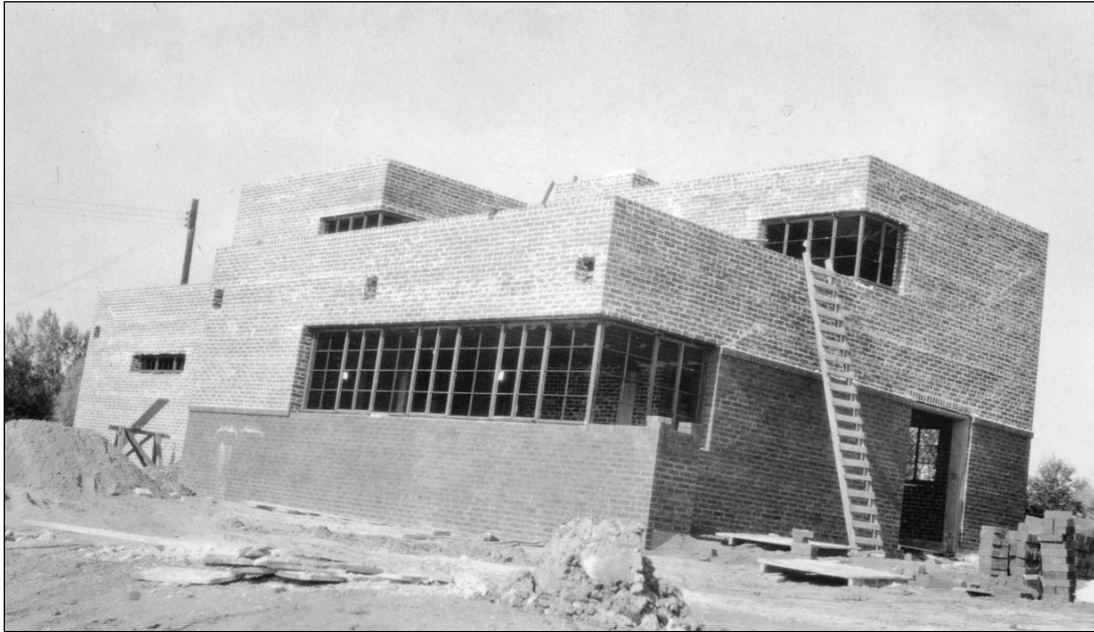
Figure 4. This 1935 construction photograph (view northwest) shows the completed brick walls and the installed steel casement windows. SOURCE: Frank Hegner photograph collection, on file Carol and Tom Amy, Denver, Colorado.
