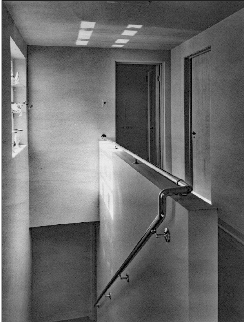
Figure 9. This ca. 1937 photograph (view west-northwest) shows the stairs to the second story with their stainless steel rail. This view appeared in Architectural Forum in April 1937. SOURCE: Frank Hegner photograph collection, on file Carol and Tom Amy, Denver, Colorado.
