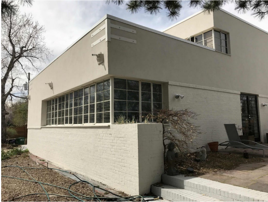
12. Long ribbon window on front and east walls of house. Photographer: Linda McVey. Date: April 2019. View northwest.
