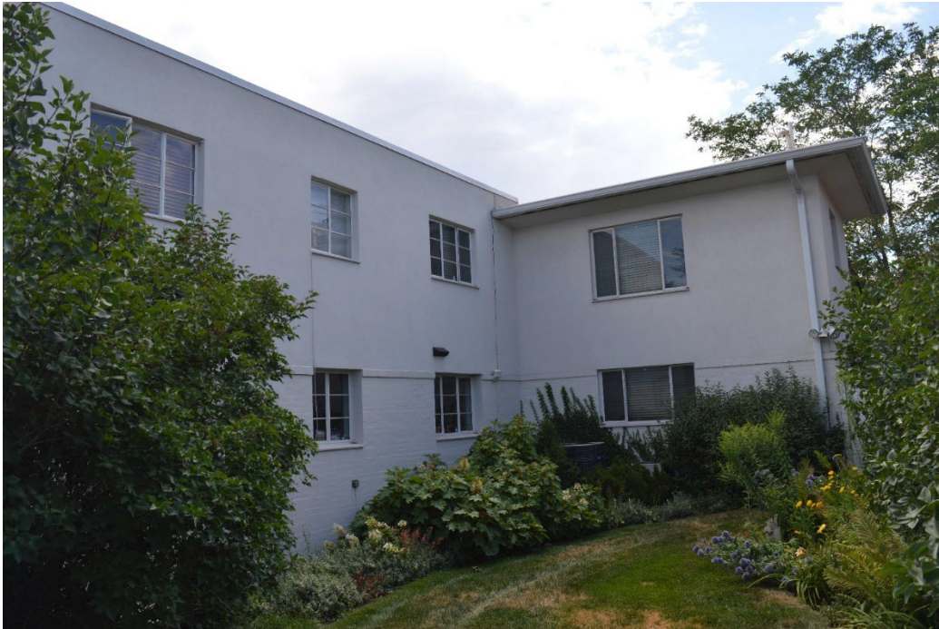
19. North wall of the 1936 section of house and east wall of the 1949 addition. Photographer: Thomas H. Simmons. Date: July 2022. View southwest.
