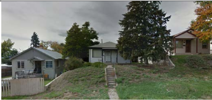
7. West across Lowell Boulevard
