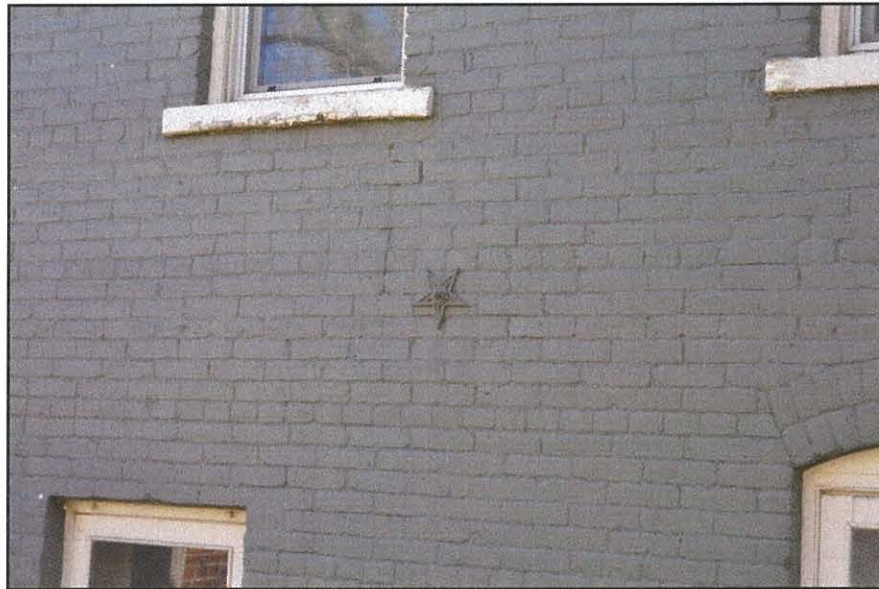
Anchor plate on west elevation
