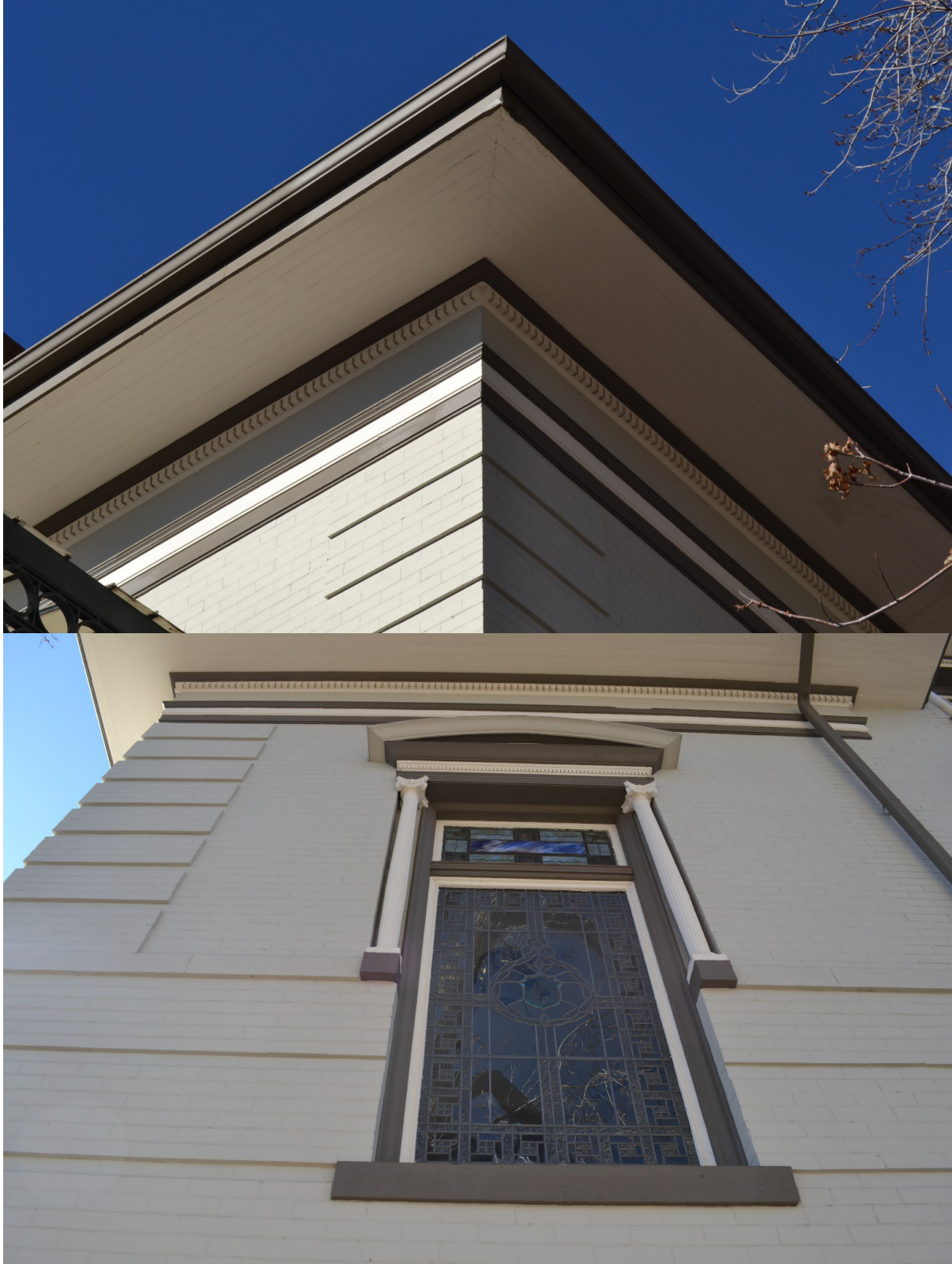
(Above) Belt Course. Pilasters around window. Dentils above window. (Below) Quoins on corners. Dentils.
