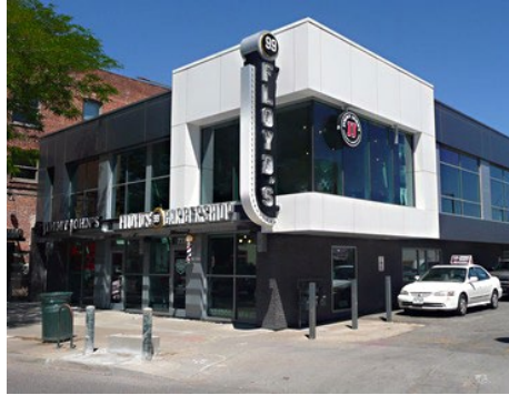
Cube Building - The Creative Farm
