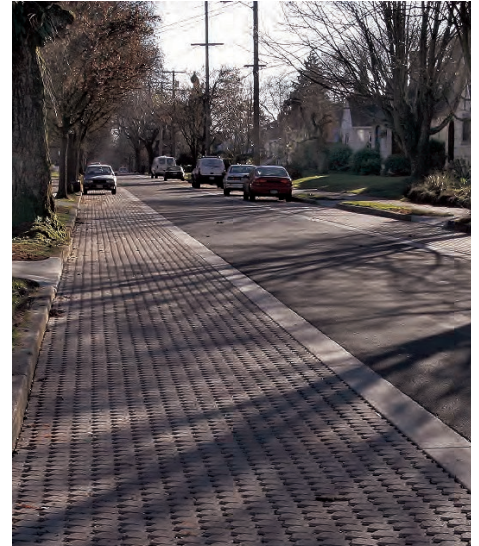
Pervious pavers for Water Quality
