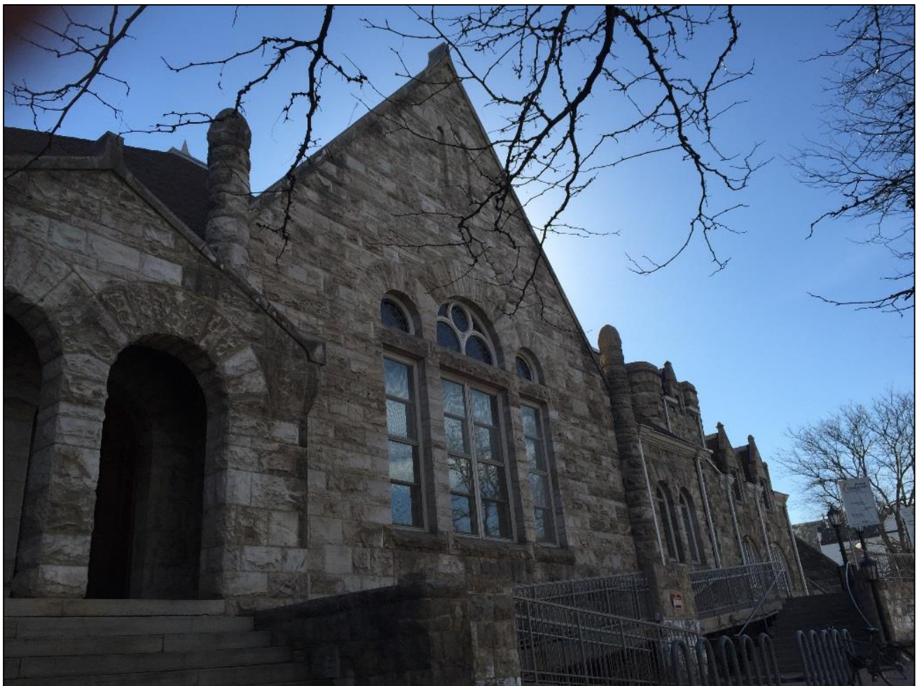
1400 Lafayette Street – First Unitarian Society of Denver, west elevation
