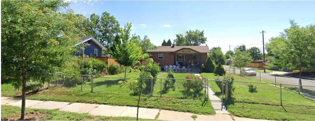
View of single unit homes south of the subject properties, looking east.
