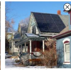
36. On a side-facing roof plane of a primary structure, minimize visual impacts by locating solar collectors on the rear 2/3 of the roof length. The collectors illustrated above do not minimize visual impacts because they are located on the front 1/3 of the roof length.
