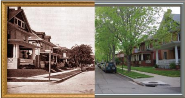
Collax Avenue A, Frank S. Snell Subdivision Historic District. Historic photo on left 1911; current photo on right 2014.
