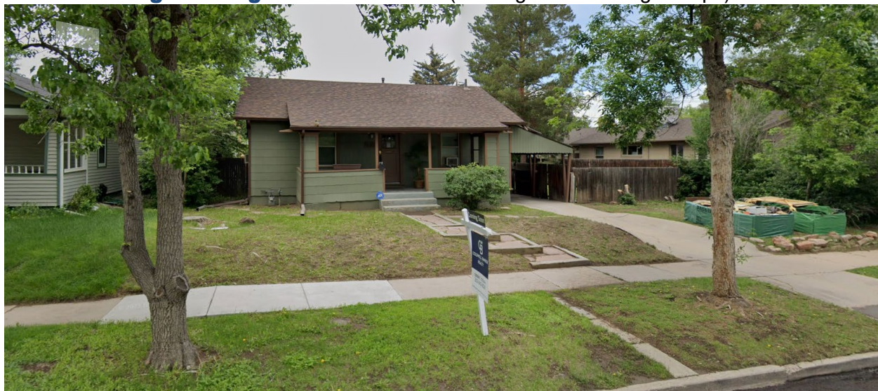
Subject Site - View of the subject property, looking west.
