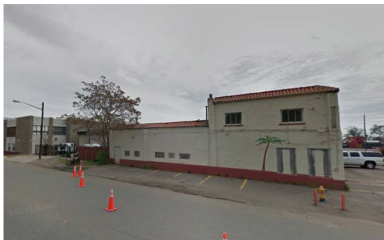
East – along Fox Street, north of 43 rd Ave. (Source: Google)
