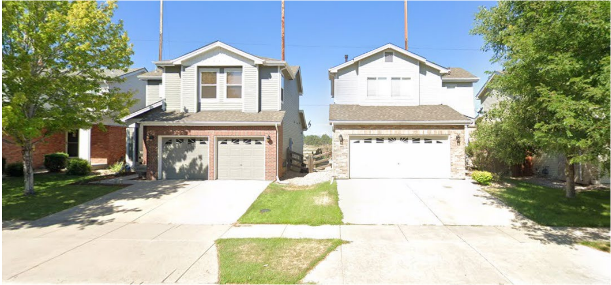
Single-unit homes directly east of the subject property, looking west.
