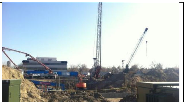
View of the adjacent property to the south from the site
