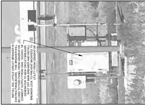
2 MIDFIELD RVR GENERATOR CONNECTION N.T.S. E-776
