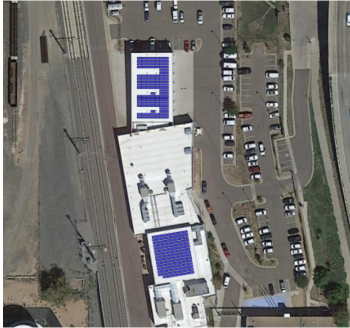
Additional PV - Police Traffic Ops Complex Bldgs
