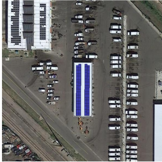
New PV on existing canopy - CPC Fleet Maintenance Bldg 5
