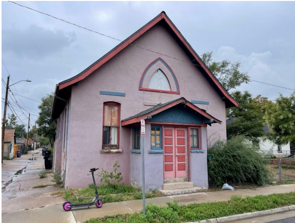
Front, north façade of church Photo provided by Historic Denver
