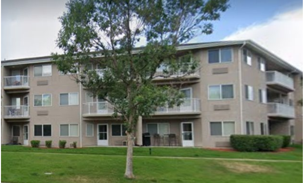
View of the property to the north looking west.
