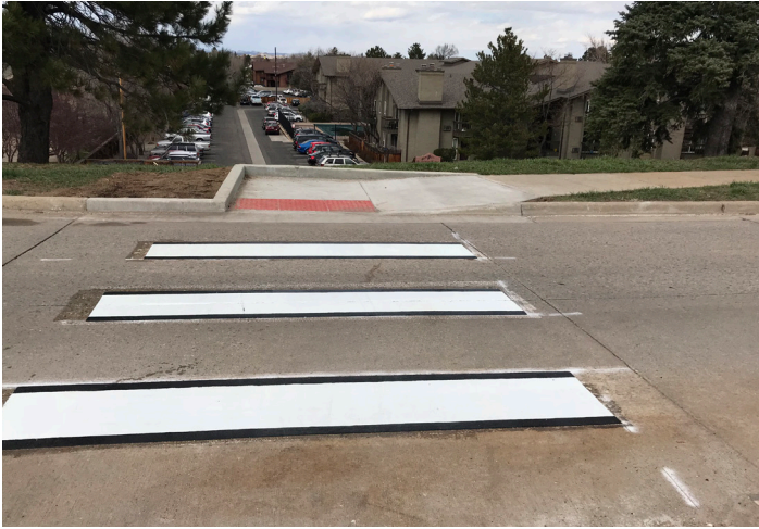
Crosswalk Pavement Marking
