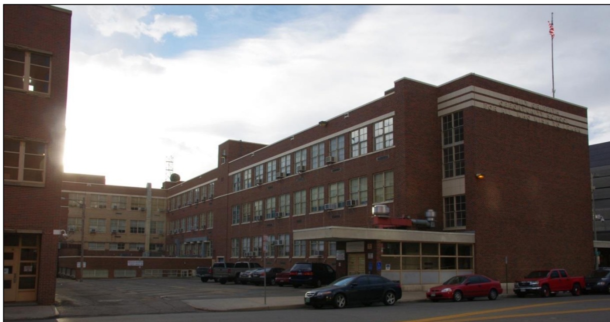
View looking northwest at the rear of the 1956 addition and its entry vestibule from 13 th Street
