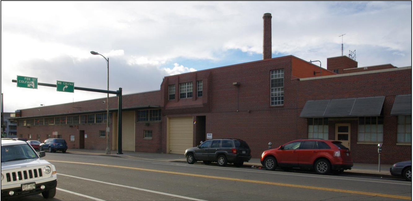
Photo, from left to right, of the 1954 Body Shop, the 1978 Auto Shop and the 1941 Shop Building on Glenarm Place. These accessory structures are located in the Non-Contributing Area of the designation.
