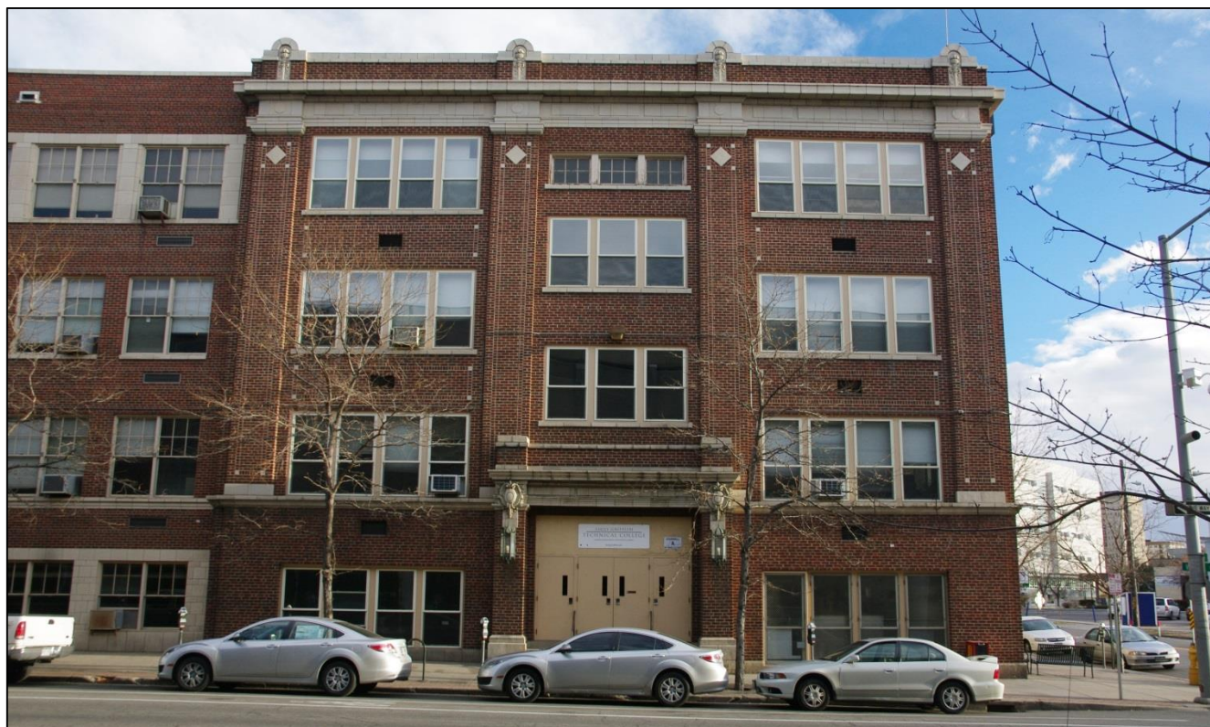
View of the Welton Street façade of the 1926 Opportunity School Building. This is the earliest building on the site and the only one dating from Emily Griffith’s tenure at the School.
