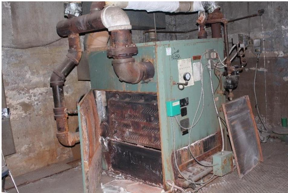
*Figure 27. Original boiler in basement/cellar.<sup>72</sup>*
