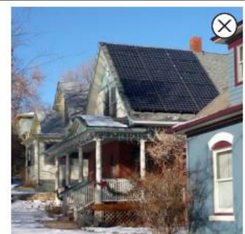
36. On a side-facing roof plane of a primary structure, minimize visual impacts by locating solar collectors on the rear 2/3 of the roof length. The collectors illustrated above do not minimize visual impacts because they are located on the front 1/3 of the roof length.
