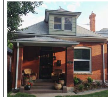
3. Simplified Classic cottage. Note the masonry porch piers, the large overhanging roof eave, the dormer window in the hipped roof, and the jack arch window
