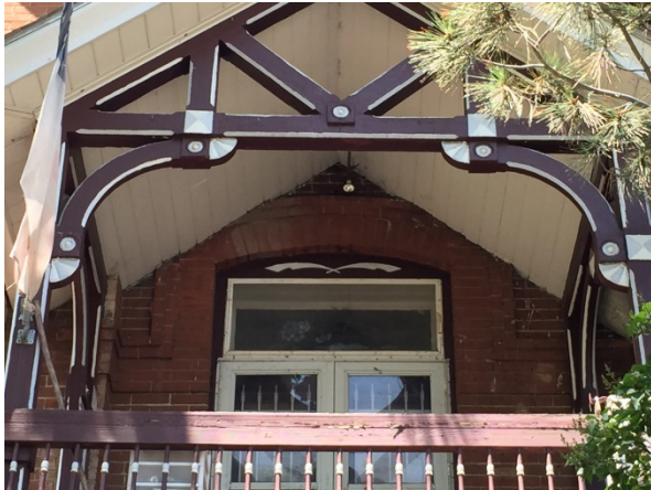
Close up view of front porch
