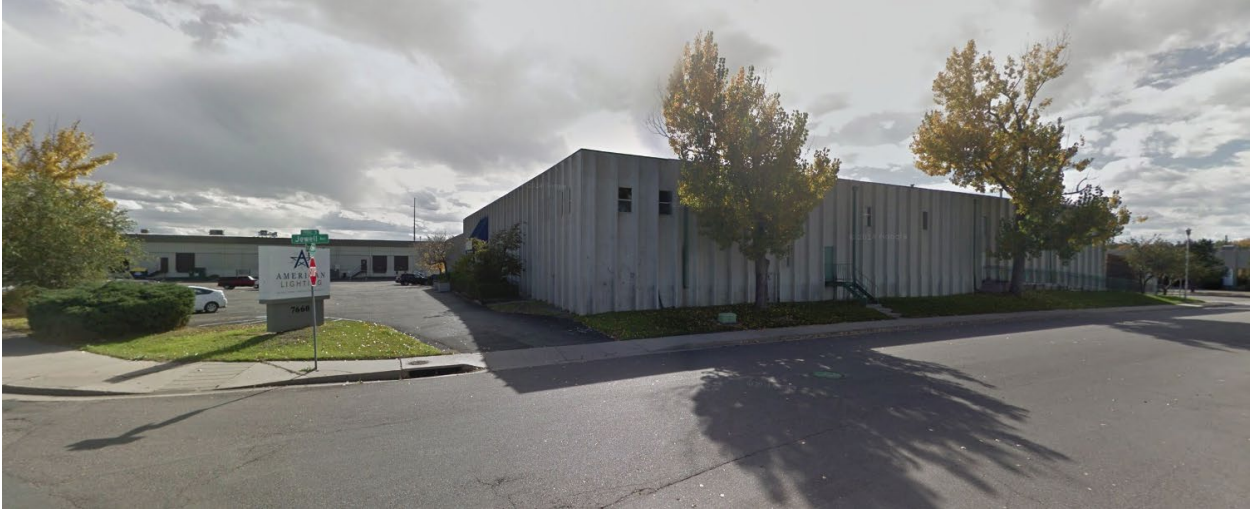
Industrial properties viewed from Jewell Avenue at Cherry Creek South Drive facing southwest
