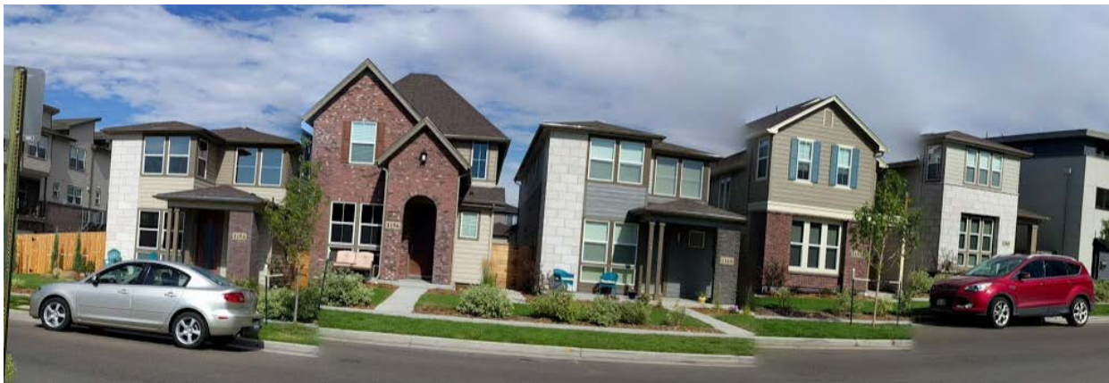
Subject site looking east.
