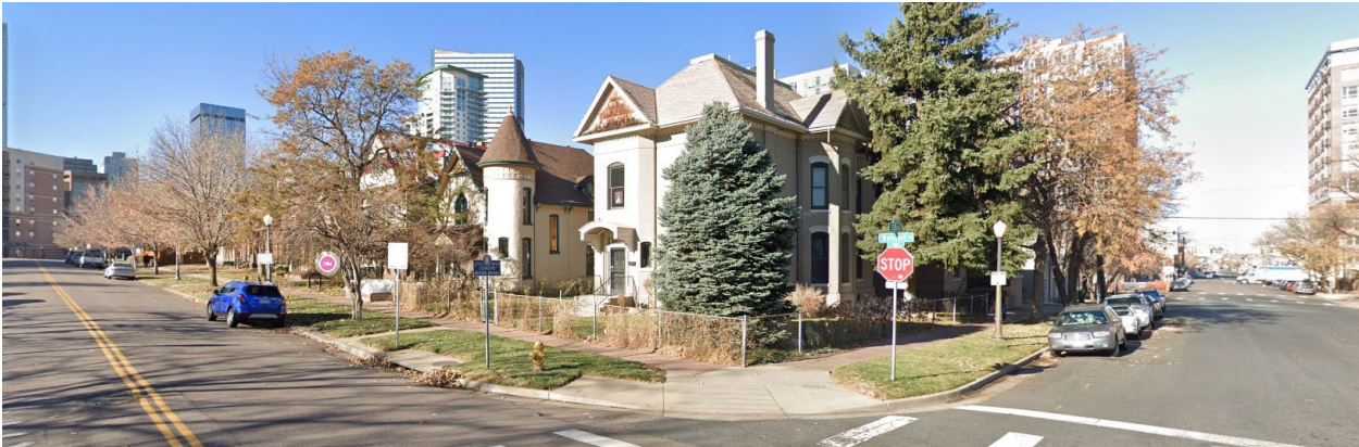
Northeast – from the corner of Tremont Place and 22 nd Street, looking west.
