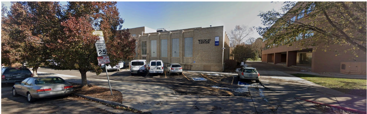
View of the property to the east, looking east.
