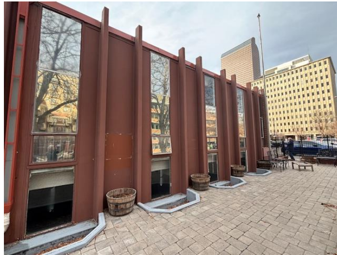
[1555 N. Grant, 1963 Event Hall east façade; note: double-tees extend both above the parapet & below the main level floor, view nw, 12.09.25]
