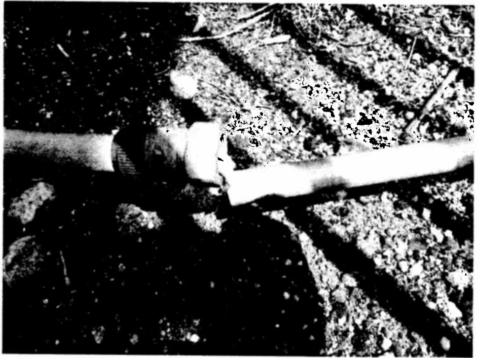
A broken electrical conduit no longer conforms to code
