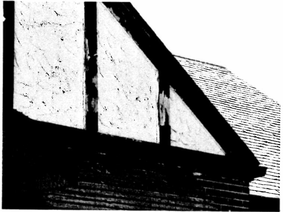
Deteriorated exterior finish
