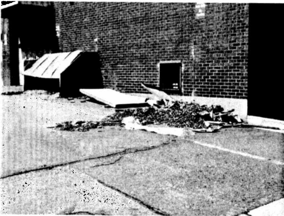
Areas that showed lack of maintenance were common
