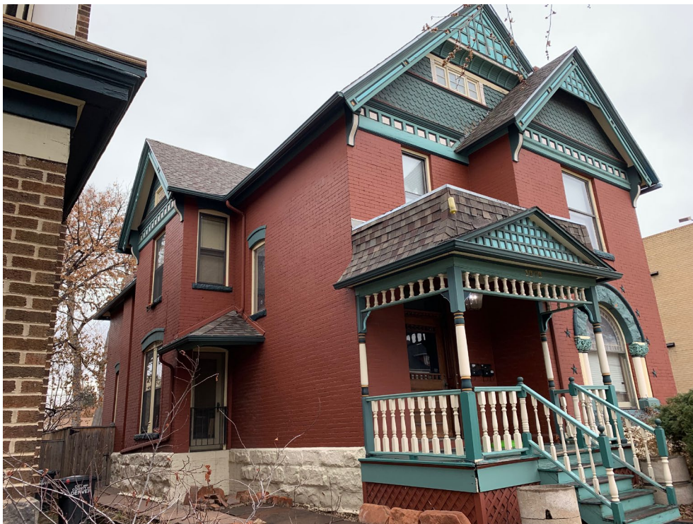
Photo 2: Northwest façade, looking southeast, Winter 2020
