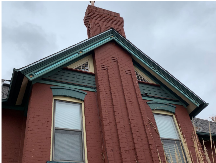
Photo 7: Chimney detail on south facade, Winter 2020
