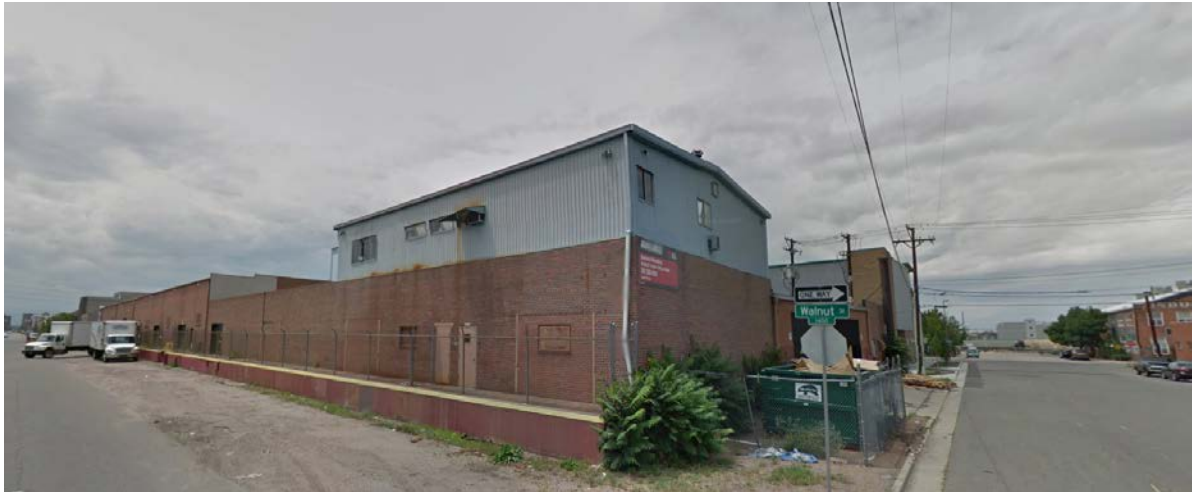
Warehouse to the northwest of the site along Walnut.
