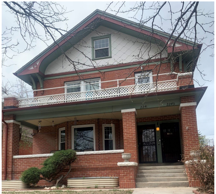
Figure 2. 2241-43 York Street front facade.
