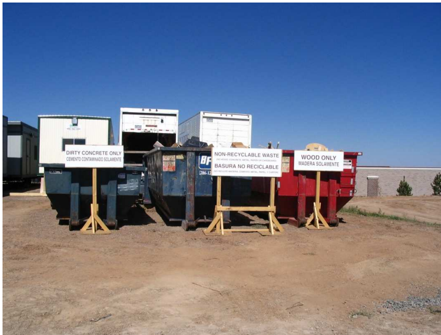
Figure 1: Dirty Concrete, Non-Recyclable Waste, and Wood Dumpsters and Signage
