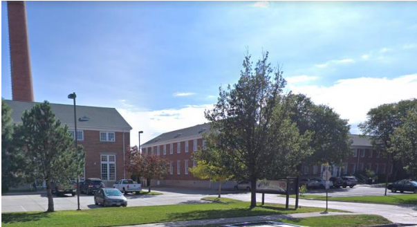
Northern portion of Subject Property
