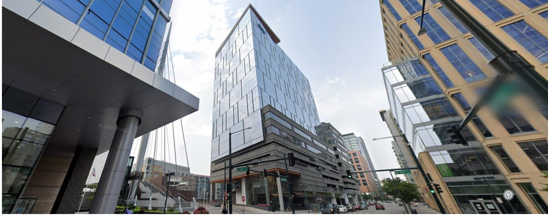
The subject property with the 19-story portion in the foreground, from Chestnut Place looking east.
