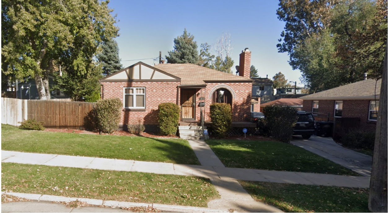
View of the property to the east.
