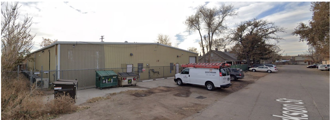
West of the subject sites, looking southeast on N. Clarkson Street.
