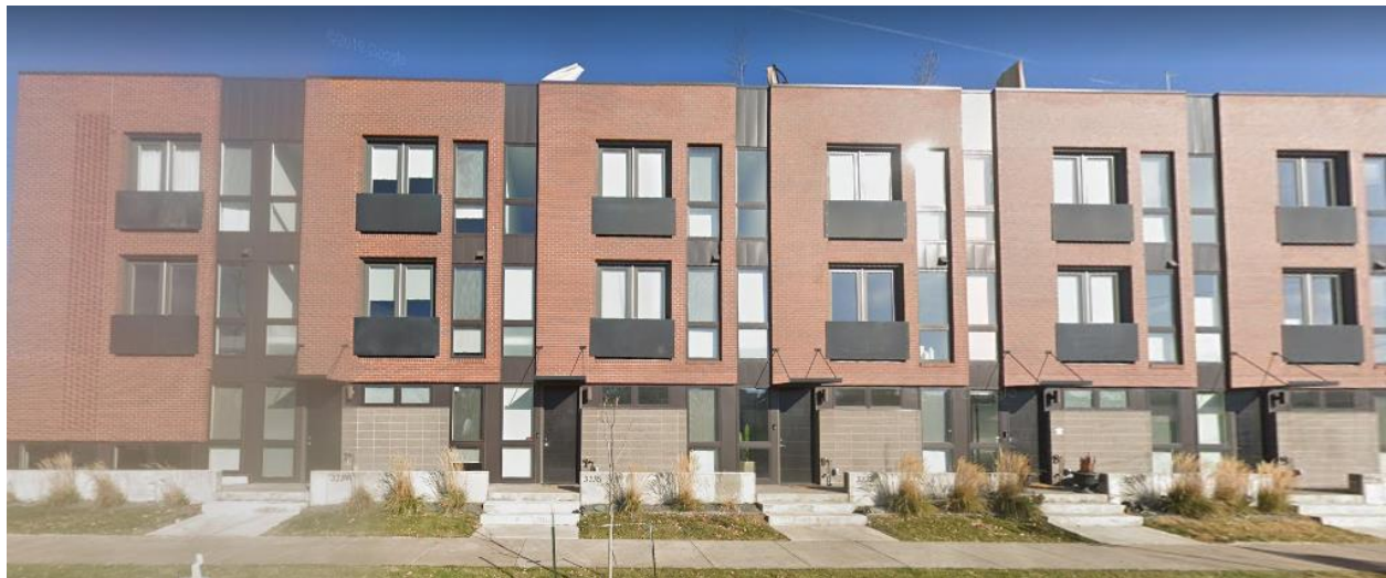
Three-story multi-unit residential building east of the subject site, facing north from 16 th Avenue.
