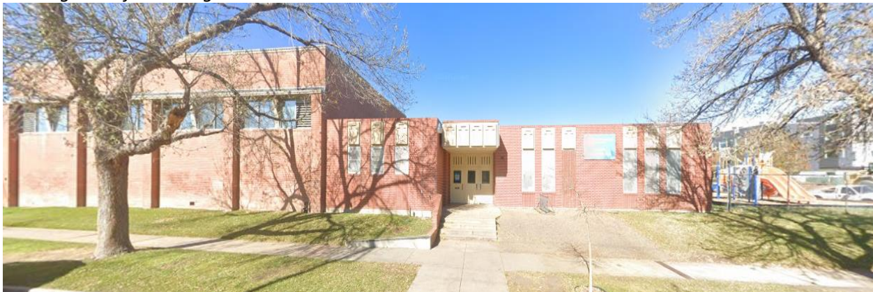
Subject property facing north from 16 th Avenue.
