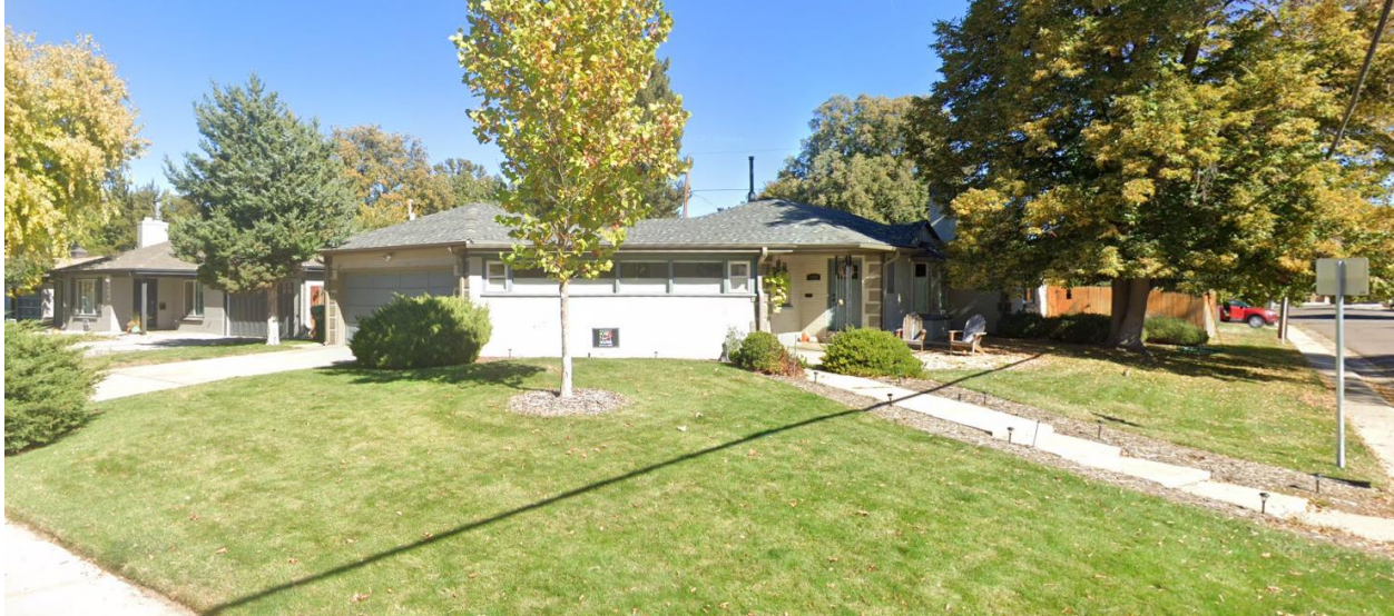
West - View of the properties to the west (on Newport St), looking northeast.
