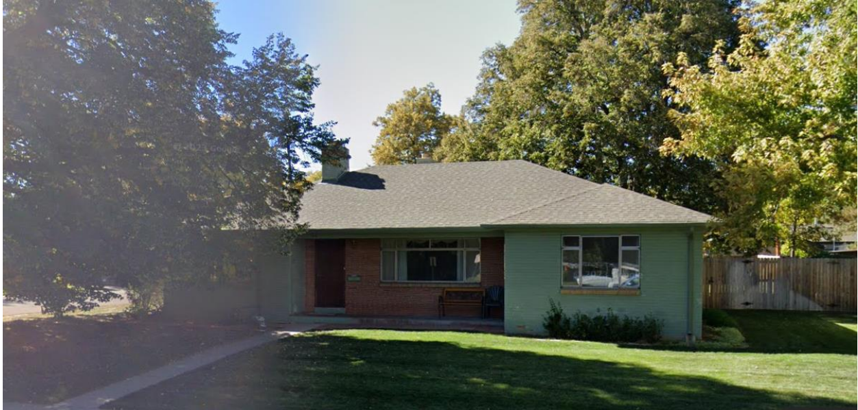
Subject Site - View of the subject property, looking west.
