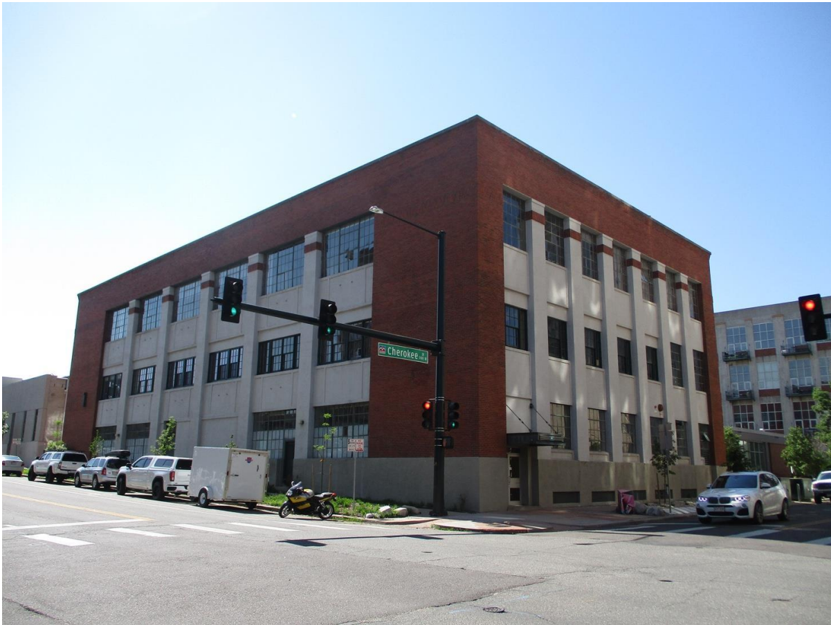
Photo of north and west elevations of Cadillac Lofts (2021)
