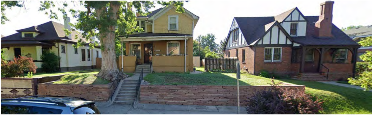
View facing east on Julian Street south of 42 nd Avenue – within proposed rezoning
