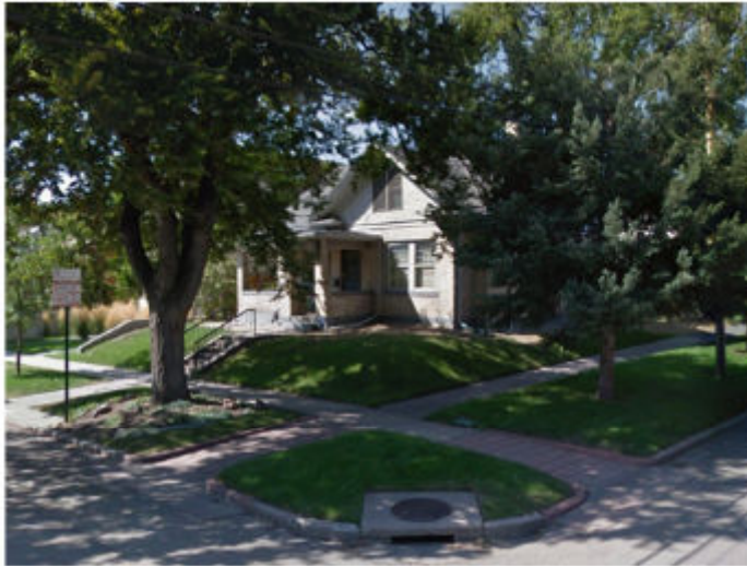
Subject Site, looking southwest
