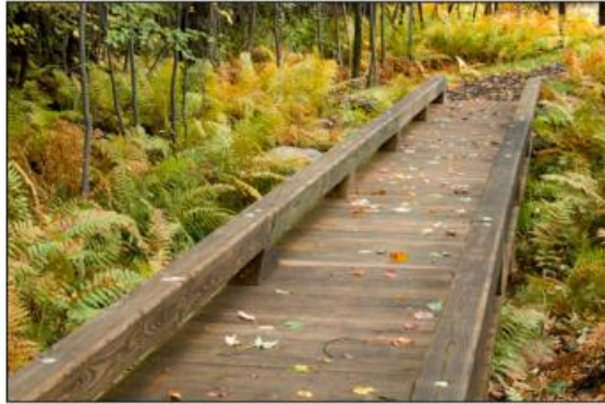
Foot Bridge (City Park hole's: 5, 6, 7)
