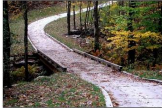
Cart Path Bridge (City Park hole's: 6, 7)
