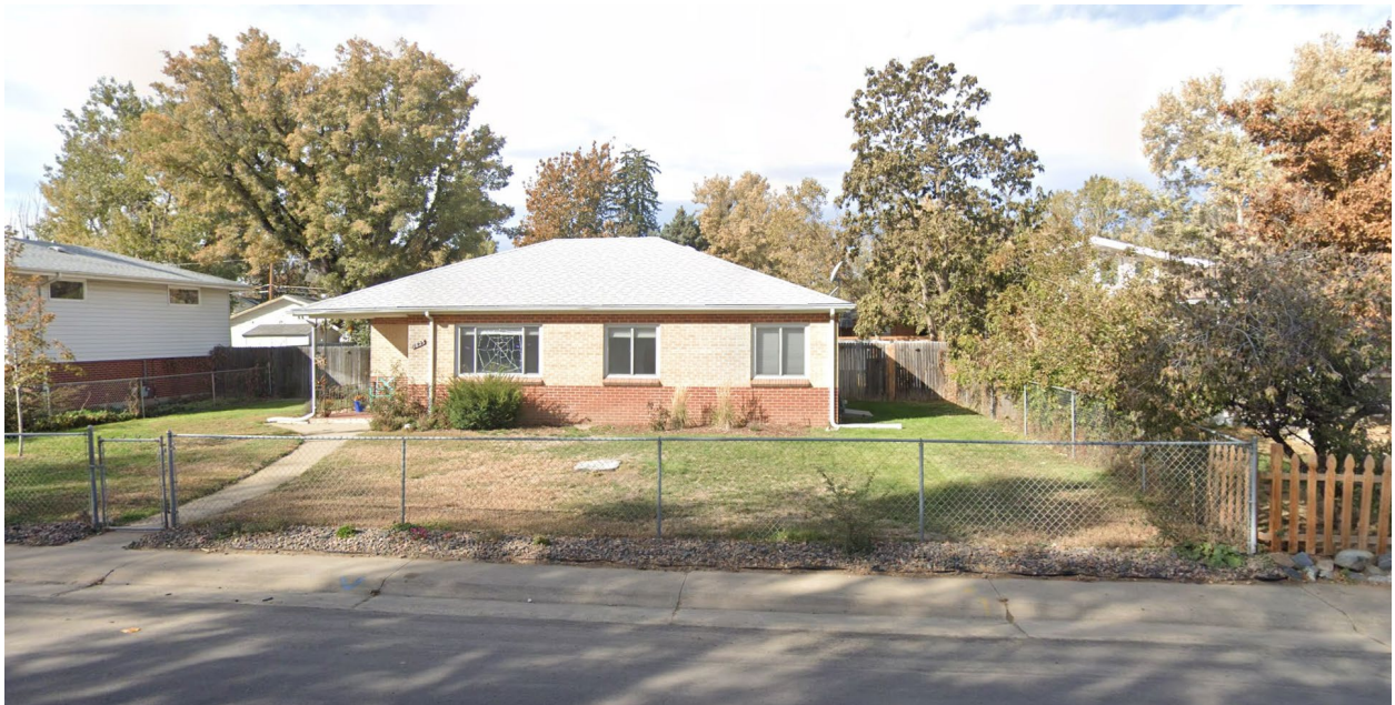
View of the property to the east.
