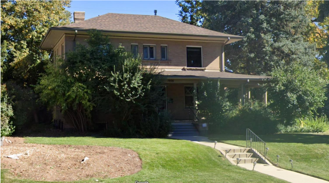
East - View of properties to the east, looking east.
