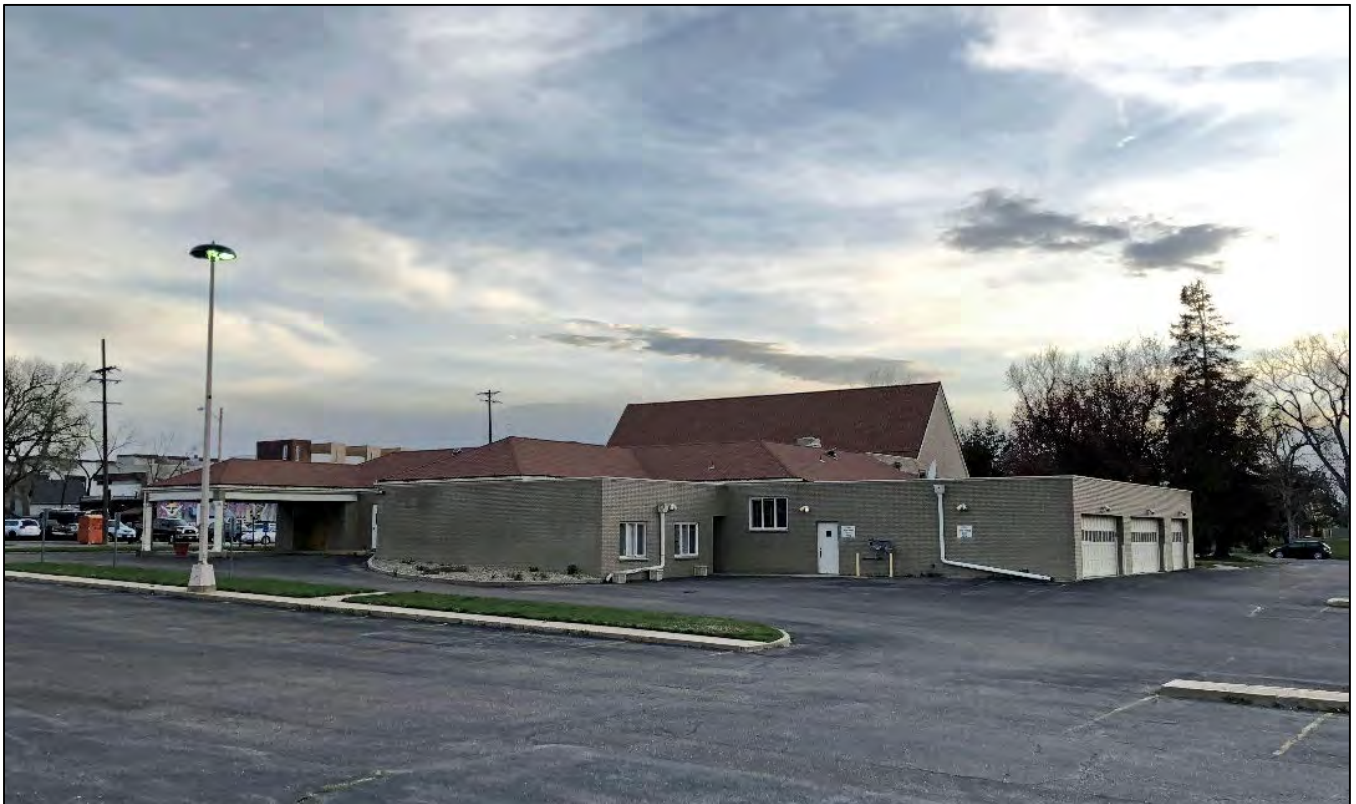
14. East wall and rear. View west-southwest, April 2018.
