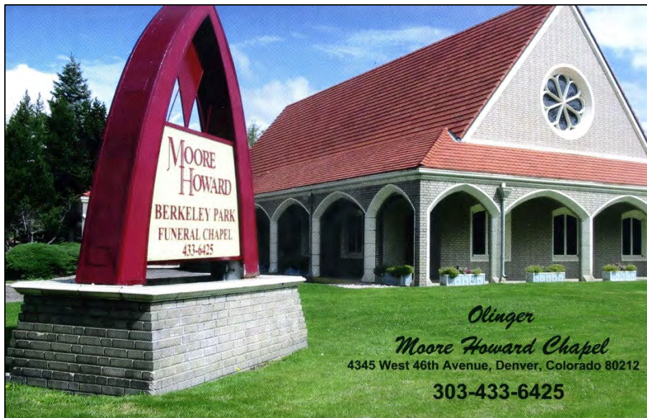
6. This ca. 2016 view northeast shows the building and the original Gothic arch freestanding sign near the southwest corner of the parcel. SOURCE: historic postcard view.
