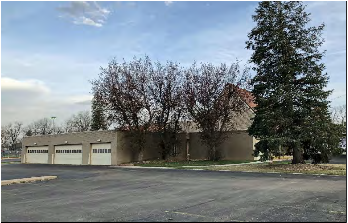
13. West end of rear. View southeast, April 2018.
