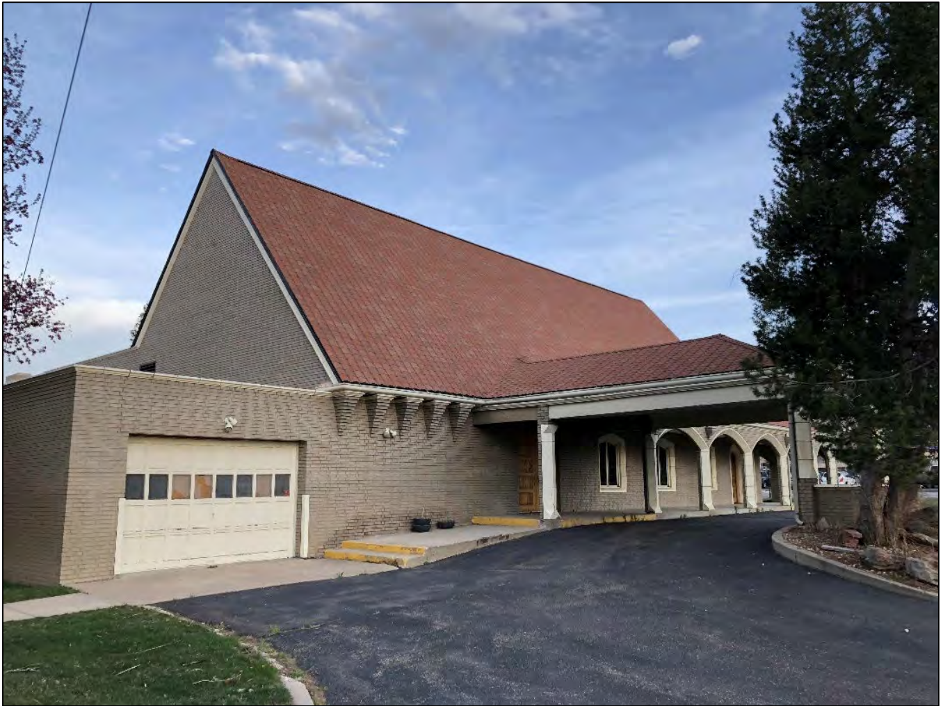
12. West wall. View southeast, April 2018.
