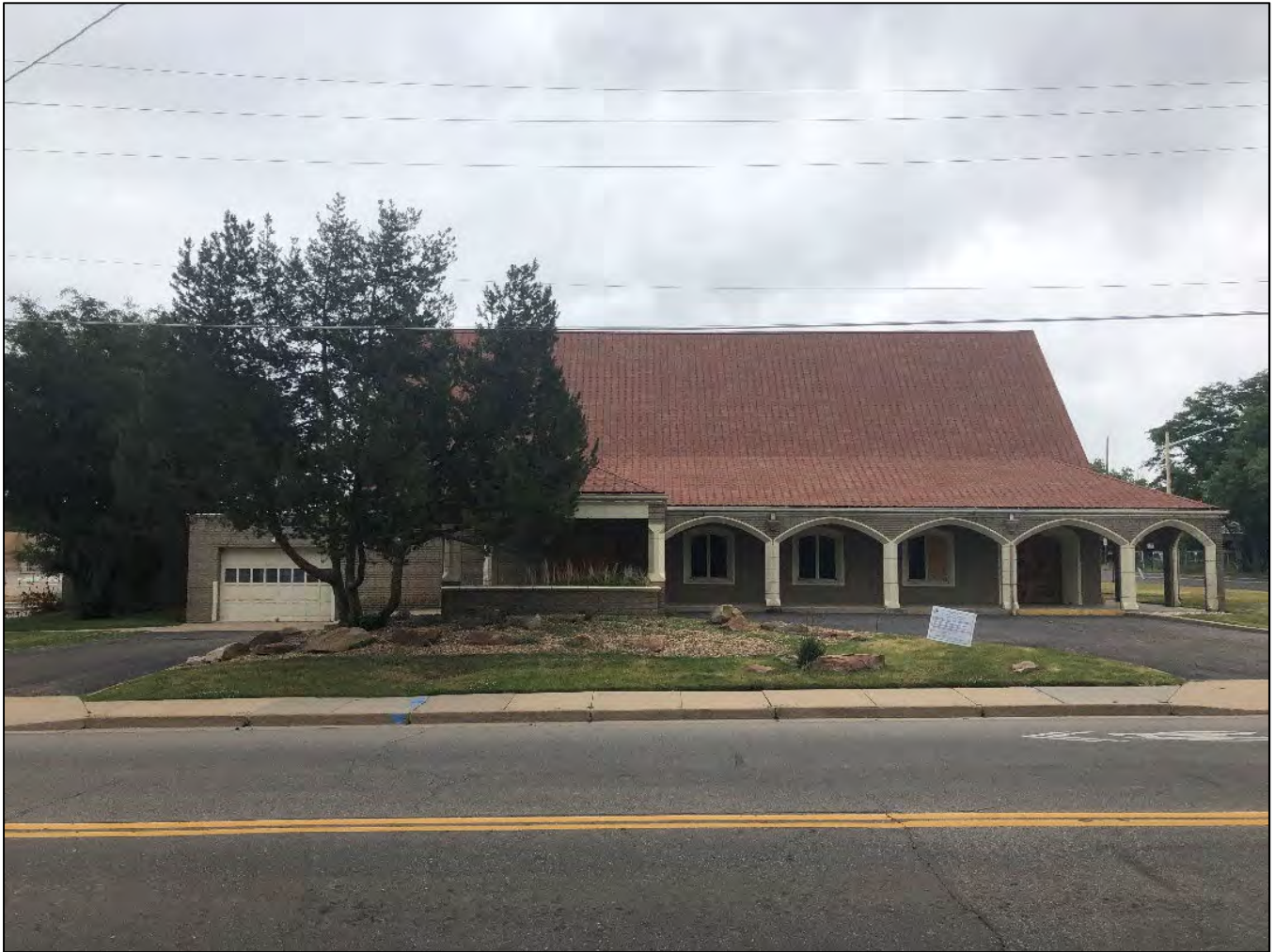
11. West wall. View east, June 2019.
