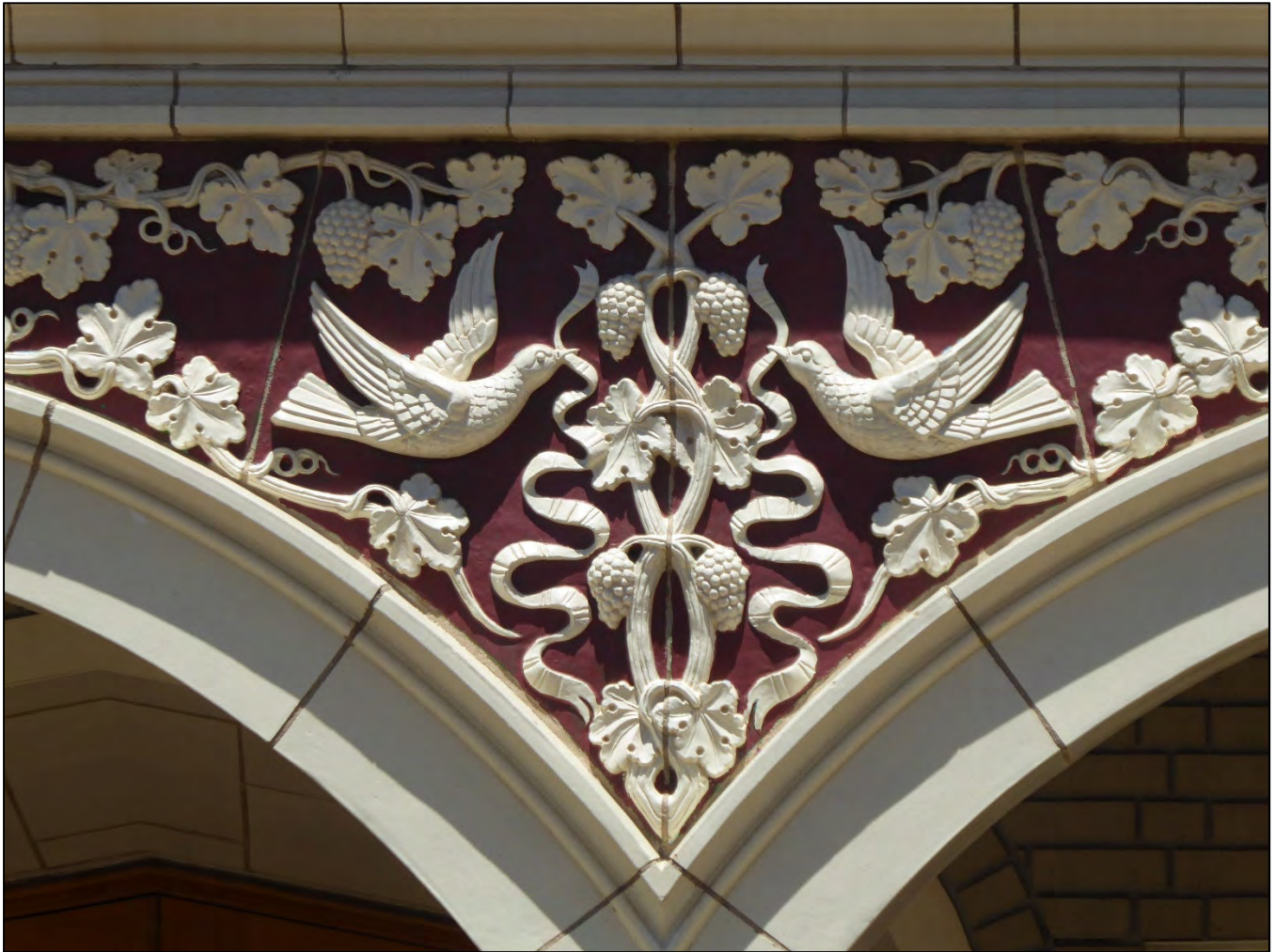
3. Portico terra cotta detail (front). View north, July 2019.
