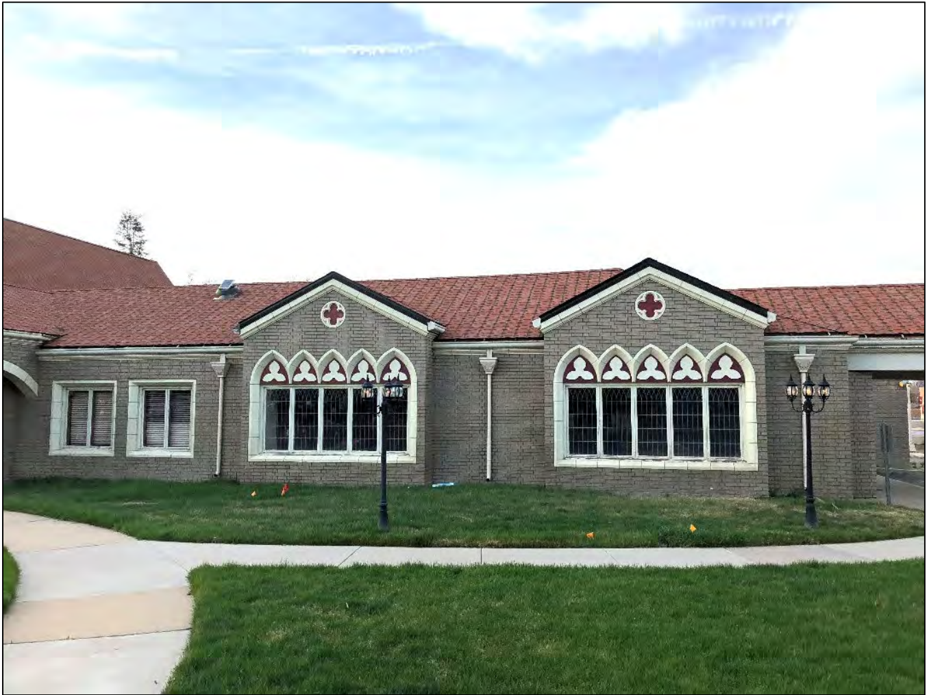
5. East end of the front. View north, April 2018.
