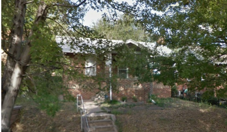
View of the property, looking west
