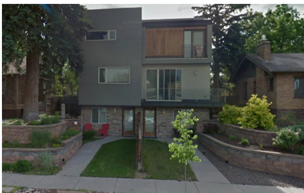
View of a neighboring property to the south, looking west
