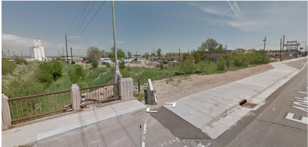
Subject site, looking northeast
